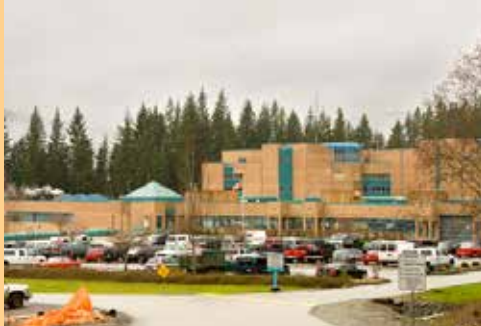
Fraser Regional Correctional Centre Maple Ridge · 253 Employees
