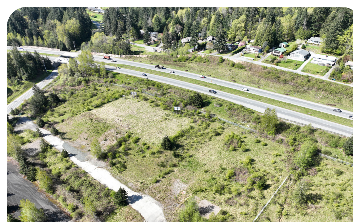
TOP OF LOWER PARCEL
